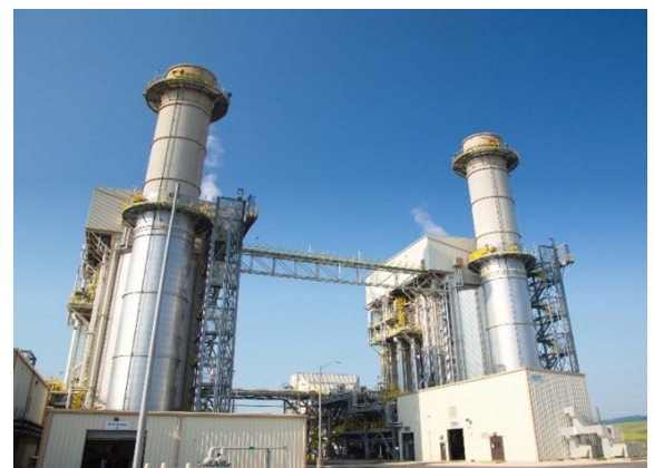
Cane Run Natural Gas Combined Generating Station in Louisville, KY. Image: OCED
