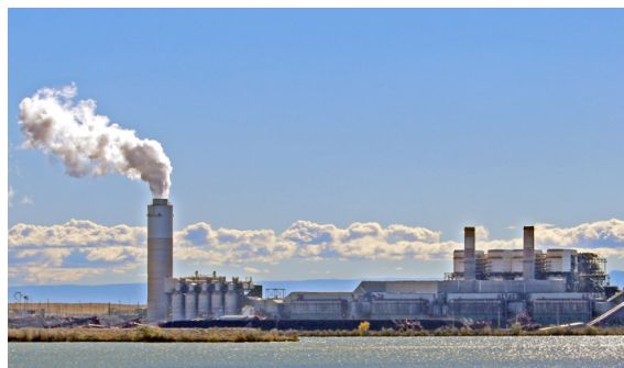
The Four Corners Power Plant located near Fruitland, NM, within the boundary of the Navajo Nation Reservation. Image: OCED
