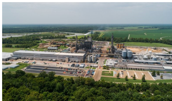
Vicksburg Containerboard Mill in Redwood, MS. Image: OCED
