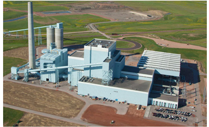
Wyoming Integrated Test Center
