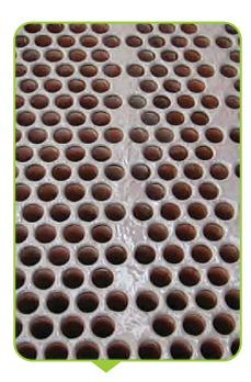
**Examples of Cleaned and Fouled Condenser Surfaces**
