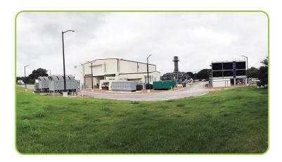
The **STEP pilot plant** will demonstrate a fully integrated, functional, electricitygenerating power plant using sCO<sub>2</sub> technology. This plant aims to show component performance and cycle operability over a range of operating conditions, as well as show progress toward a lower cost of electricity.
