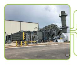
Primary heater included a hot section fabricated using IN 740H.
