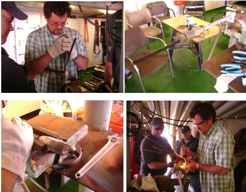
Figure 2: Cable termination on the ship's coaxial cable for piston coring lead by Ross Downer (Milbar-Hydrotest Inc.).
