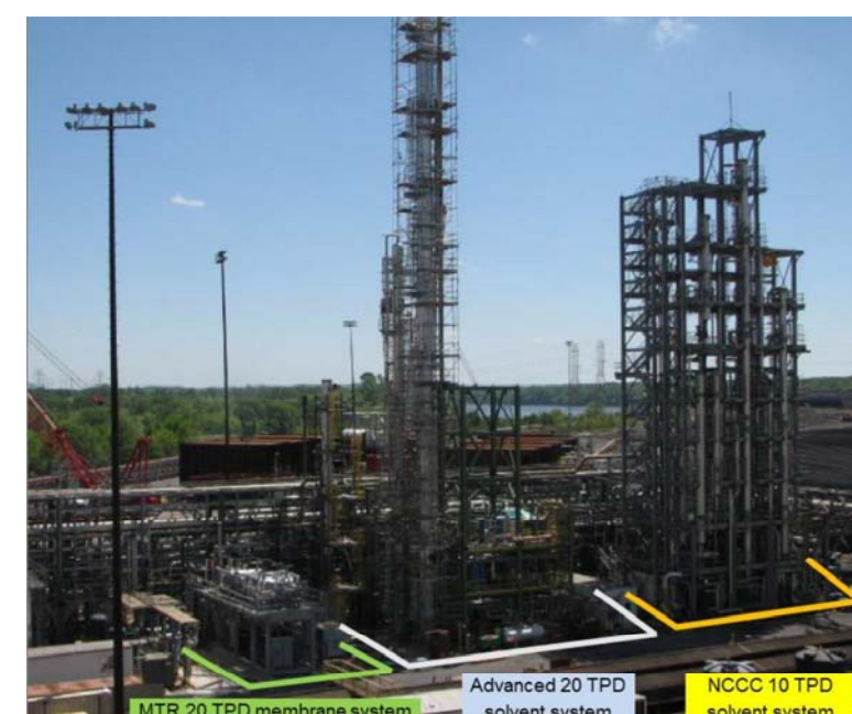
20 ton/day CO 2 capture experimental membrane system installed by MTR, Inc. at the National Carbon Capture Center. 3
