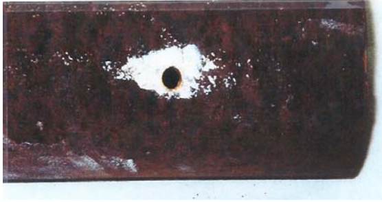
Figure 1. Pipe Showing Complete Removal of Spackling Compound
