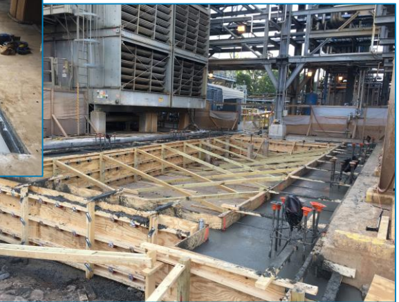
Pile caps and grade beams poured
