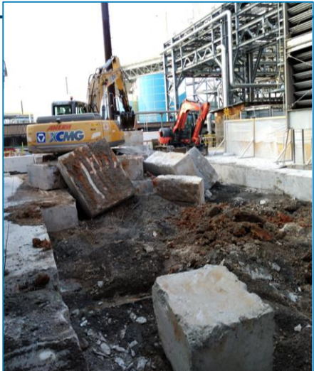
Concrete removal in progress
