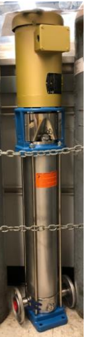
Vertical multistage centrifugal pump
