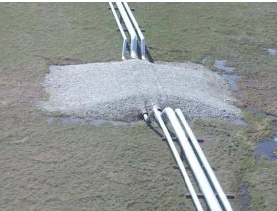
View of the pipeline crossing with protective gravel cover
