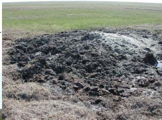
*Whitish material on mounds is excess backfill sand for leg holes, used during summer remediation to top fill leg holes showing any settlement*
