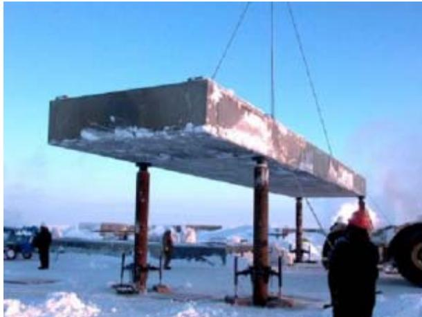
Figure E-3. Setting the First Platform Module
