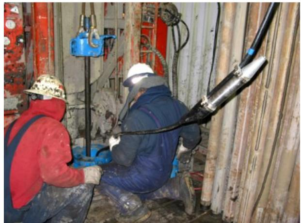
Figure E-10. Deploying VSP Array into Well
