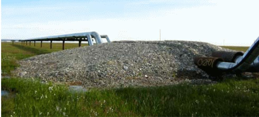
Figure 8. Gravel Ramp for Pipeline Crossing
