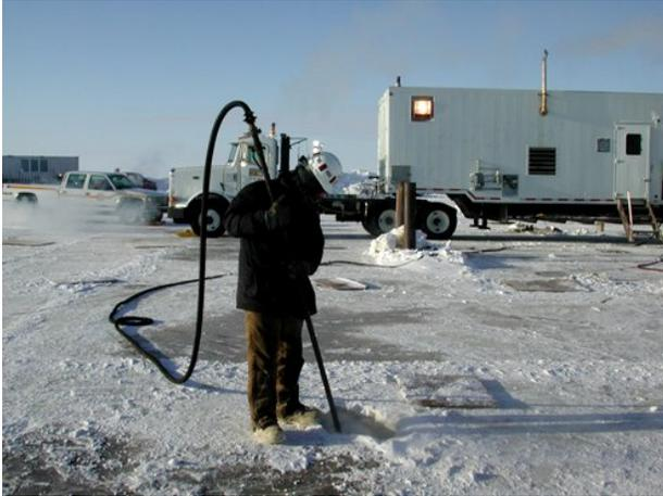
Figure E-13. Vacuuming Platform Leg Holes
