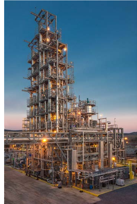
PSTU, NCCC, Wilsonville, AL (Courtesy of NCCC)
