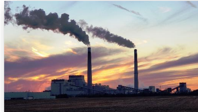
Sherburne County Generating Station, "Sherco" (Becker, MN)
