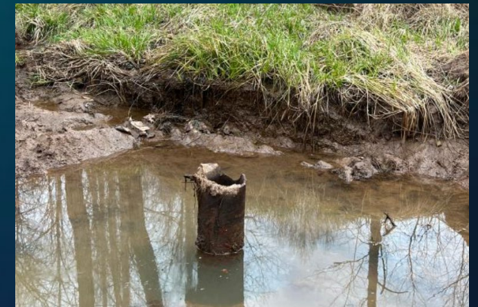
An orphaned well in WV before plugging
