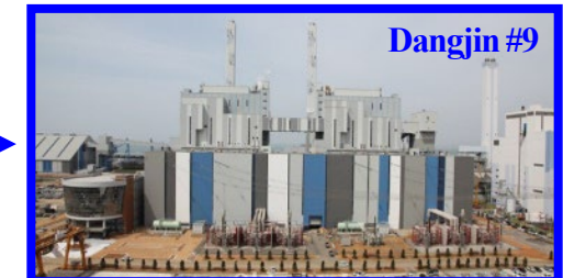
Pulverized coal - 20% NH 3 co-firing
