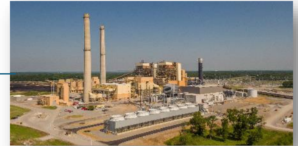
Grand River Energy Center - Thermal 520 MW Coal-Fired 495 MW Combined-Cycle Natural Gas 426 MW Simple Cycle
