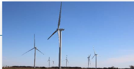
Wind Generation 385 MW Across Four Projects
