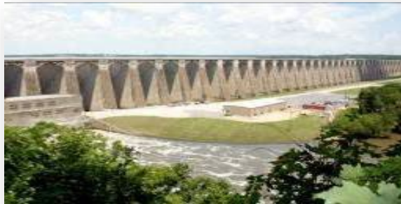
Pensacola Dam Grand Lake o' the Cherokees 126 MW Hydropower
