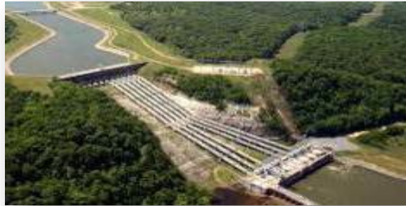
Salina Pumped Storage Project W.R. Holway Reservoir 260 MW Hydropower
