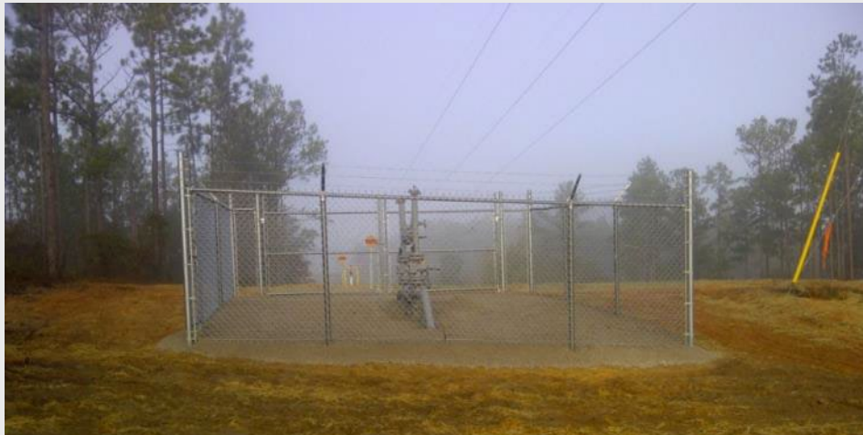
Mainline valve station along pipeline
