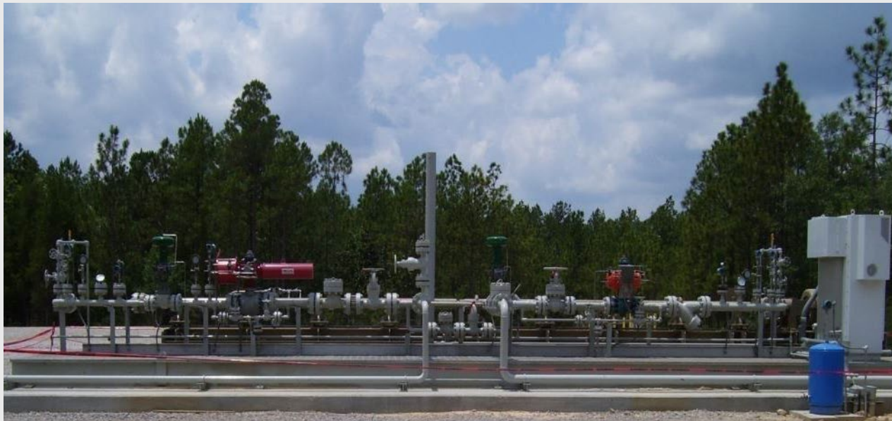
Horizontal CO 2 booster pump at D-9-7 #2 wellsite
