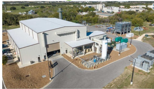
A high tech supercritical carbon dioxide power plant is taking shape behind the walls of a modern building in Texas, with the potential to lower the cost of concentrating solar power systems.
