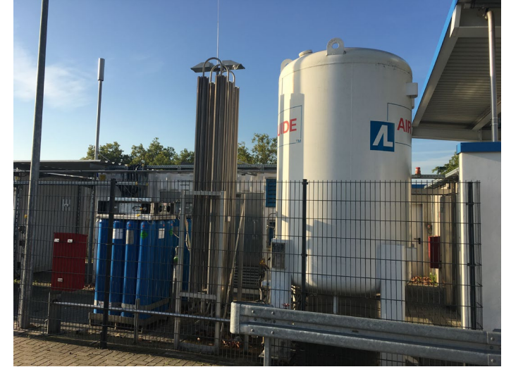
Hydrogen would be stored in 700-bar hydrogen storage tanks at the Food Distribution Center. The tanks have a similar safety profile to gasoline storage at gas stations.
