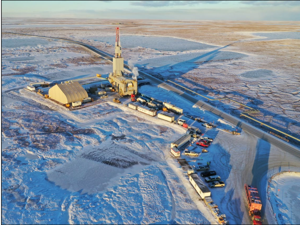
October 2022 – Drilling Operations
