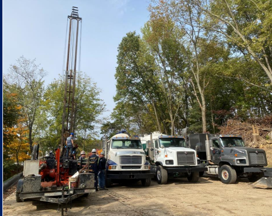
Muse Well #1 (top) Cementing (bottom)
