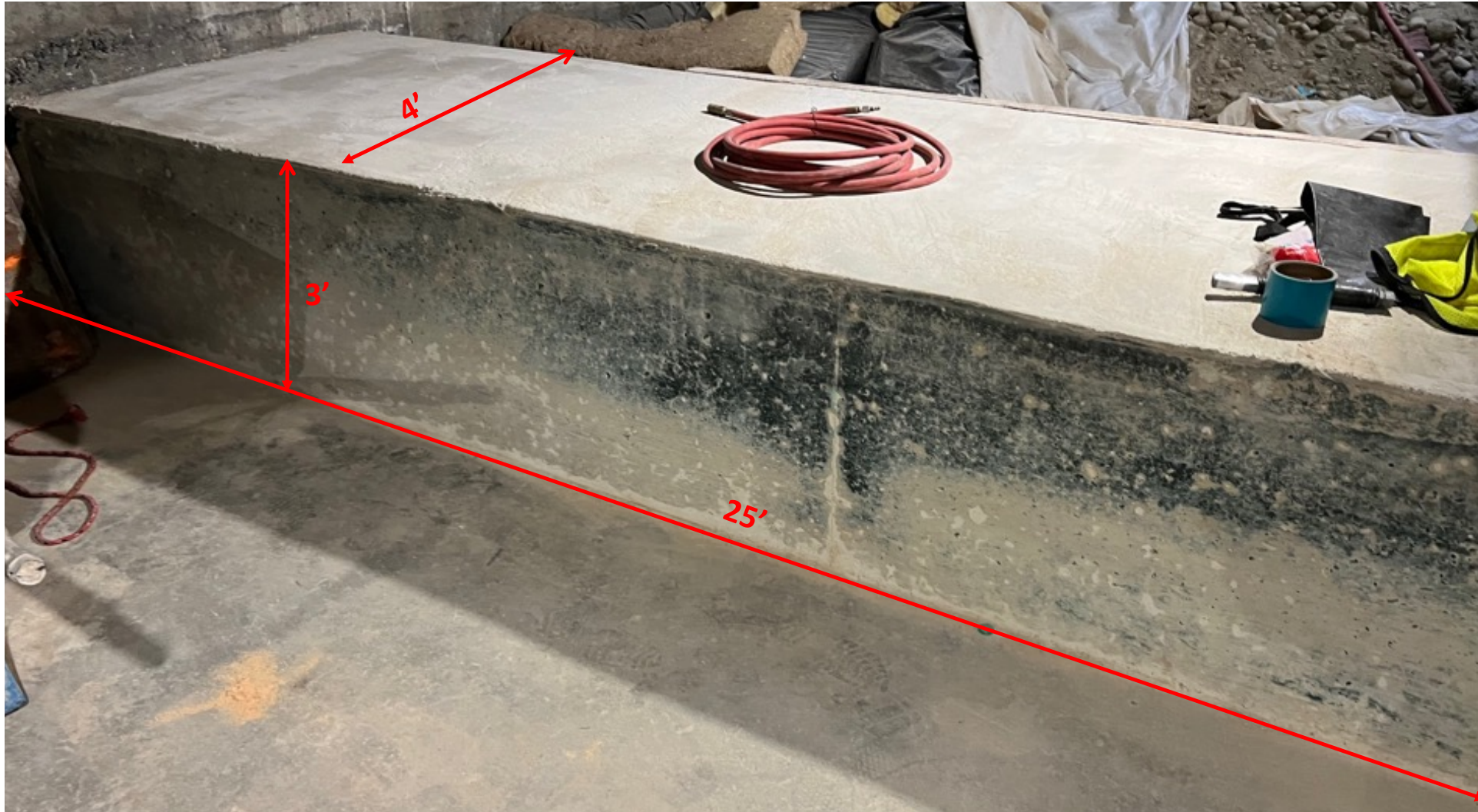
One of the foundations after demolding
