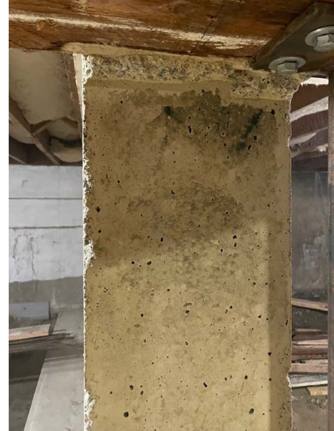
Side view of shear walls
