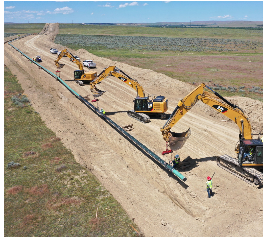
35 miles of pipeline from Douglas to Casper Wyoming
