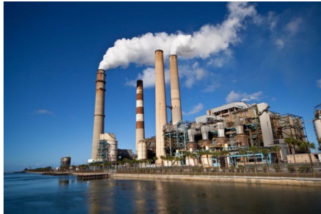
Flue Gas Capture
