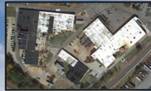
Kings Mountain, NC Plant Full Life-cycle Management
