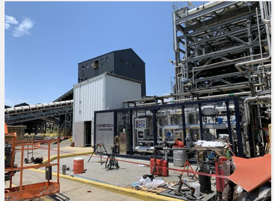
Installation currently in progress!
