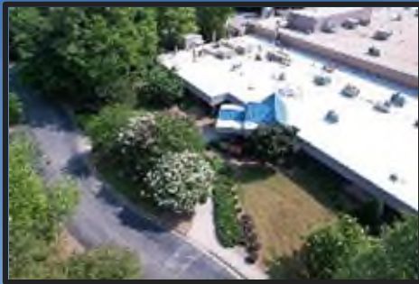
Durham, NC Plant
