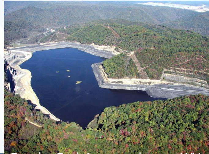
Brushy Fork impoundment, WV 31,000,000 m 3 of coal waste
