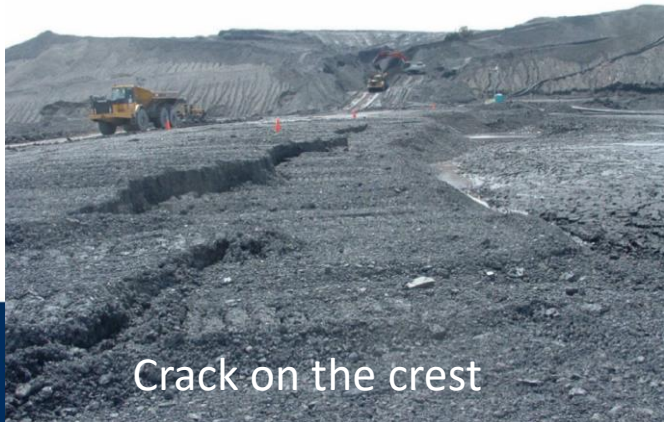
Cracks on embankment slope
