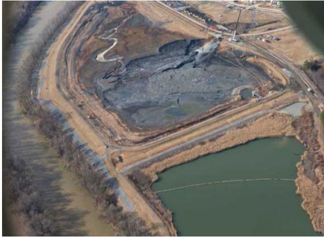
Dan River Steam Station (NC), Feb. 2014
