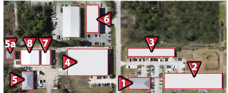
1 - ENGINEERING OFFICES 4 - PRODUCTION 6 - CONTROLLED-ATMOSPHERE BRAZING FACILITY 2 - RESEARCH & DEVELOPMENT 5 - PRODUCT DEVELOPMENT 7 - SHEET METAL FABRICATION 3 - RESEARCH & DEVELOPMENT 5a - MAINSTREAM EBEAM 8 - ROTOMOLD PRODUCTION
