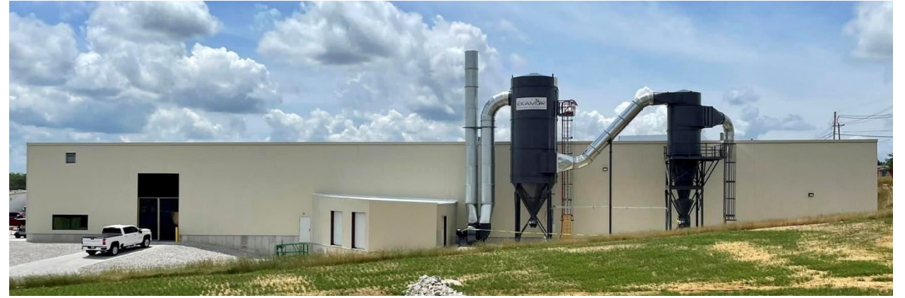
Ekamor Facility in Cookeville, TN
