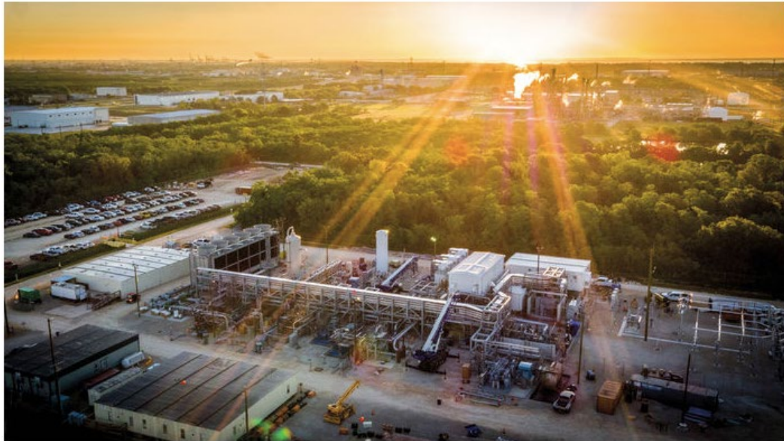
The prototype NET Power plant near Houston, Texas, is testing an emission-free technology designed to compete with conventional fossil power.
