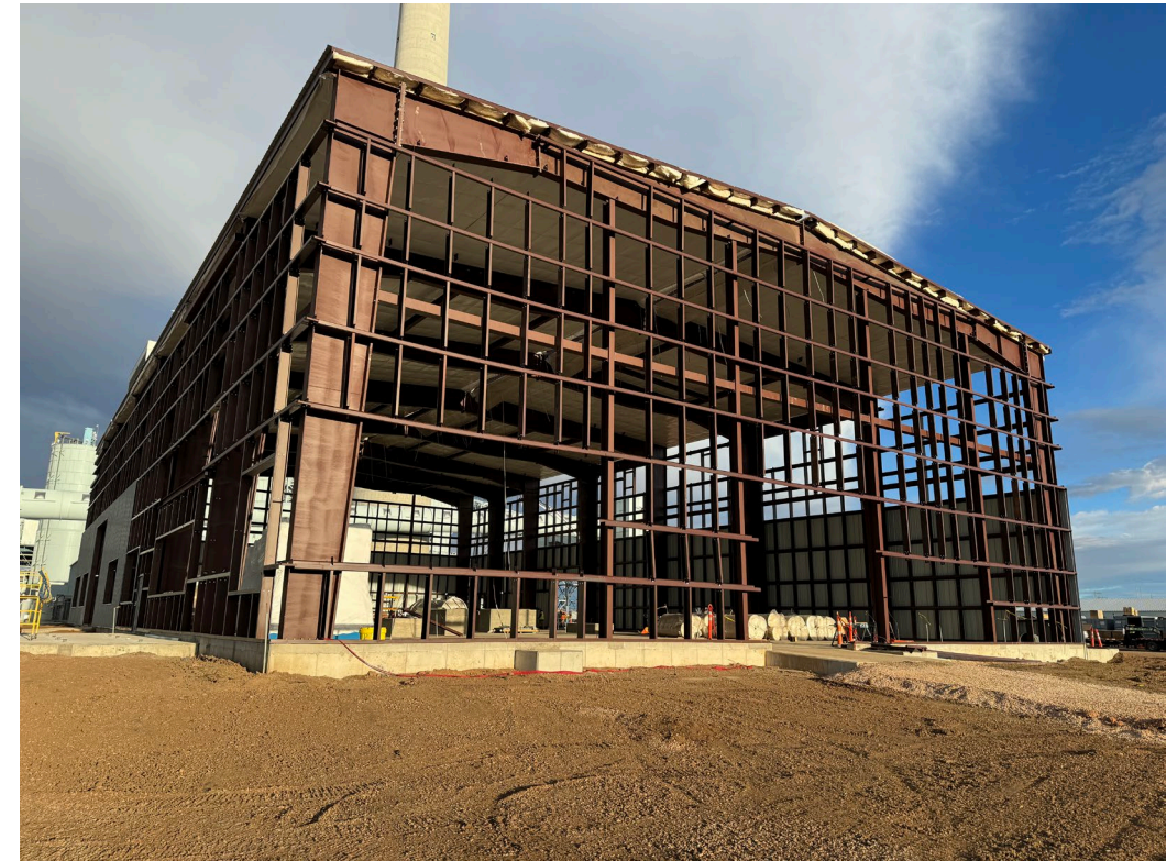
Building to house MTR system.
