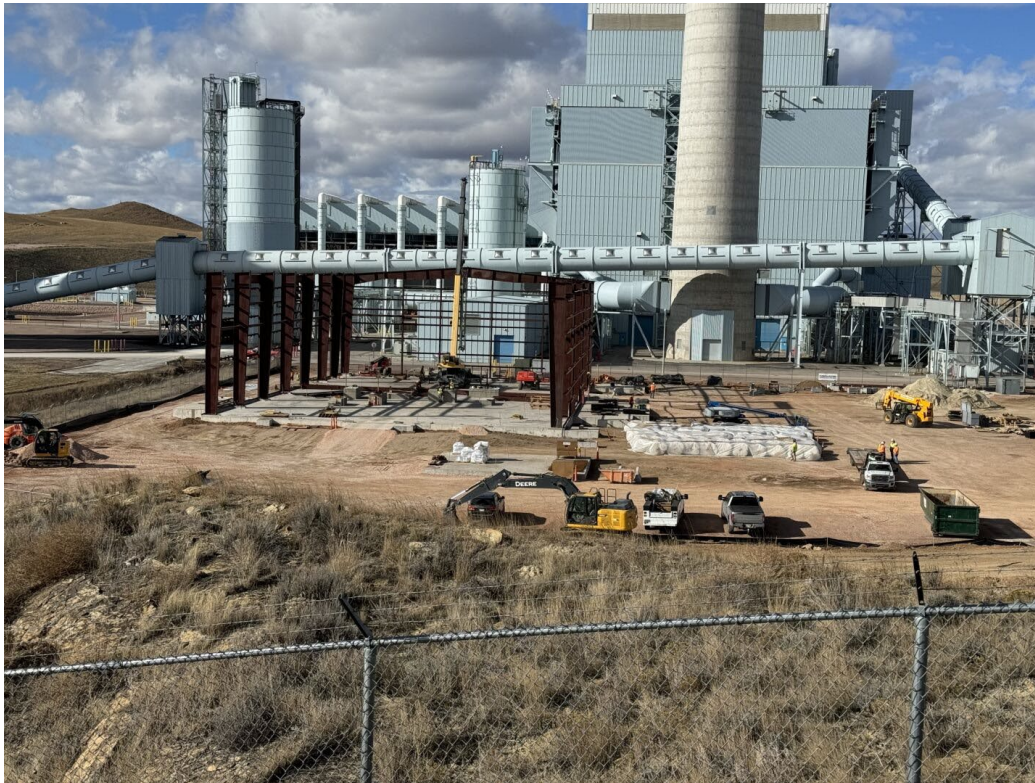
Fall of 2023 civil and structural work.
