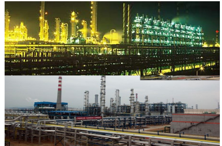
Yangtzi Petro-chemical Plant
