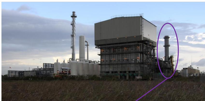
SMR Flue Gas Stack
