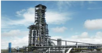
Corpus Christi, Texas - 2Mt HBI capacity connected to low cost nat gas
