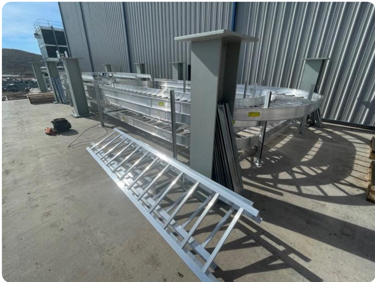
Electrical cable trays and piers for the PDC building
