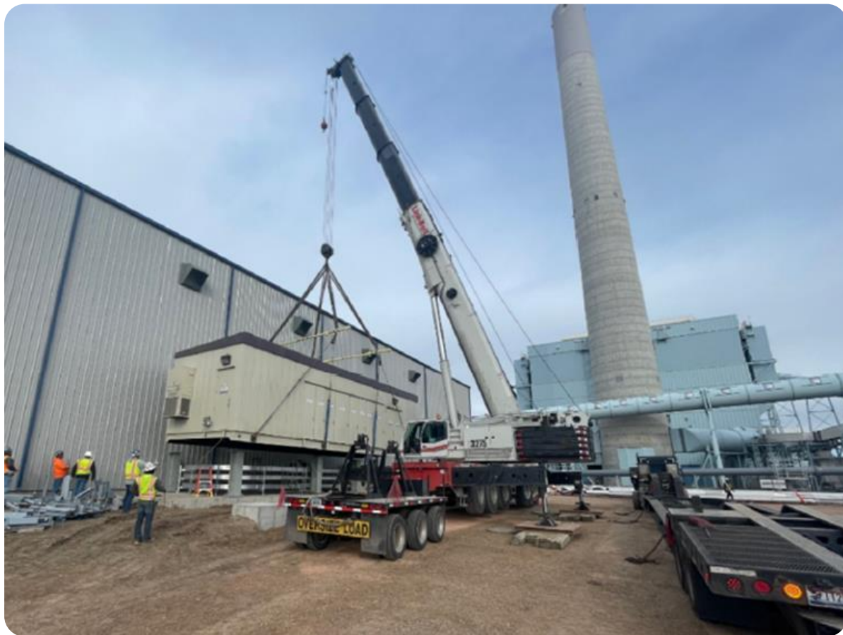
Placement of PDC building
