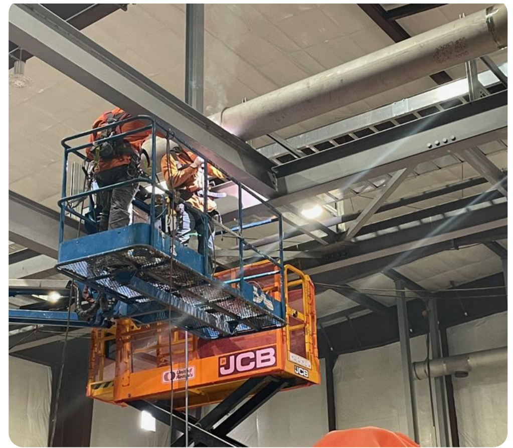
Installing process piping
