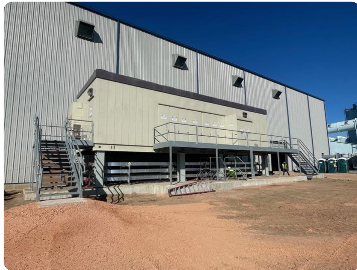
PDC building installed with stairs and walkways
