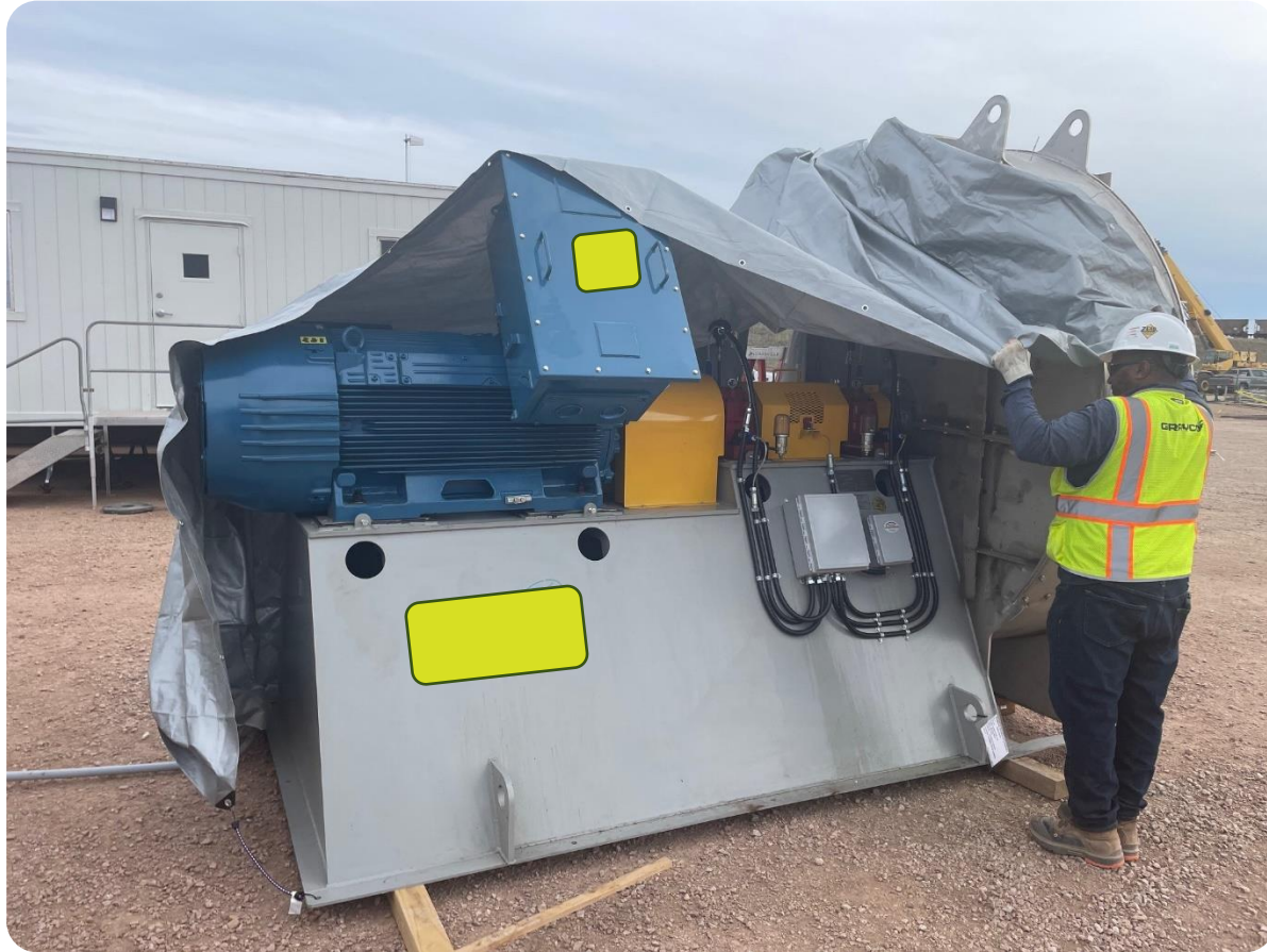
Process Equipment arrives – Flue gas blower
