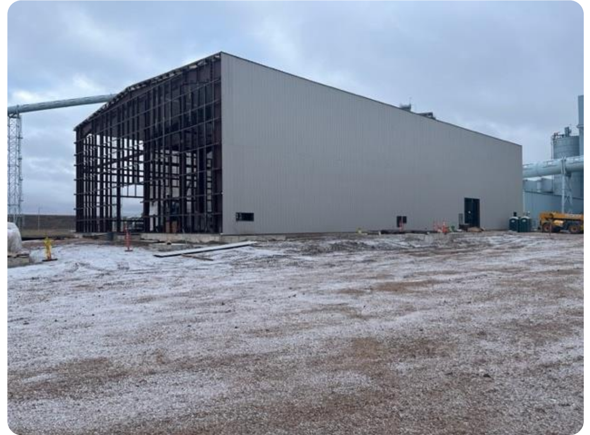
Large Pilot Capture Building
