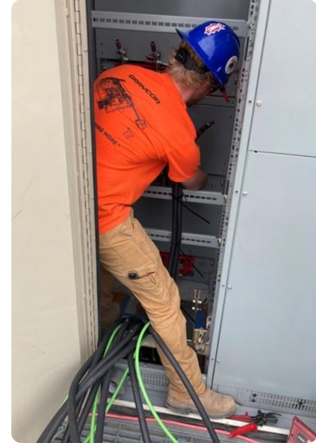
Electricians terminating cables
