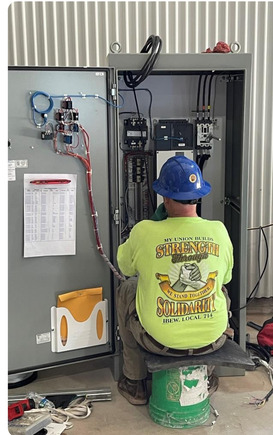
Electricians terminating cables
