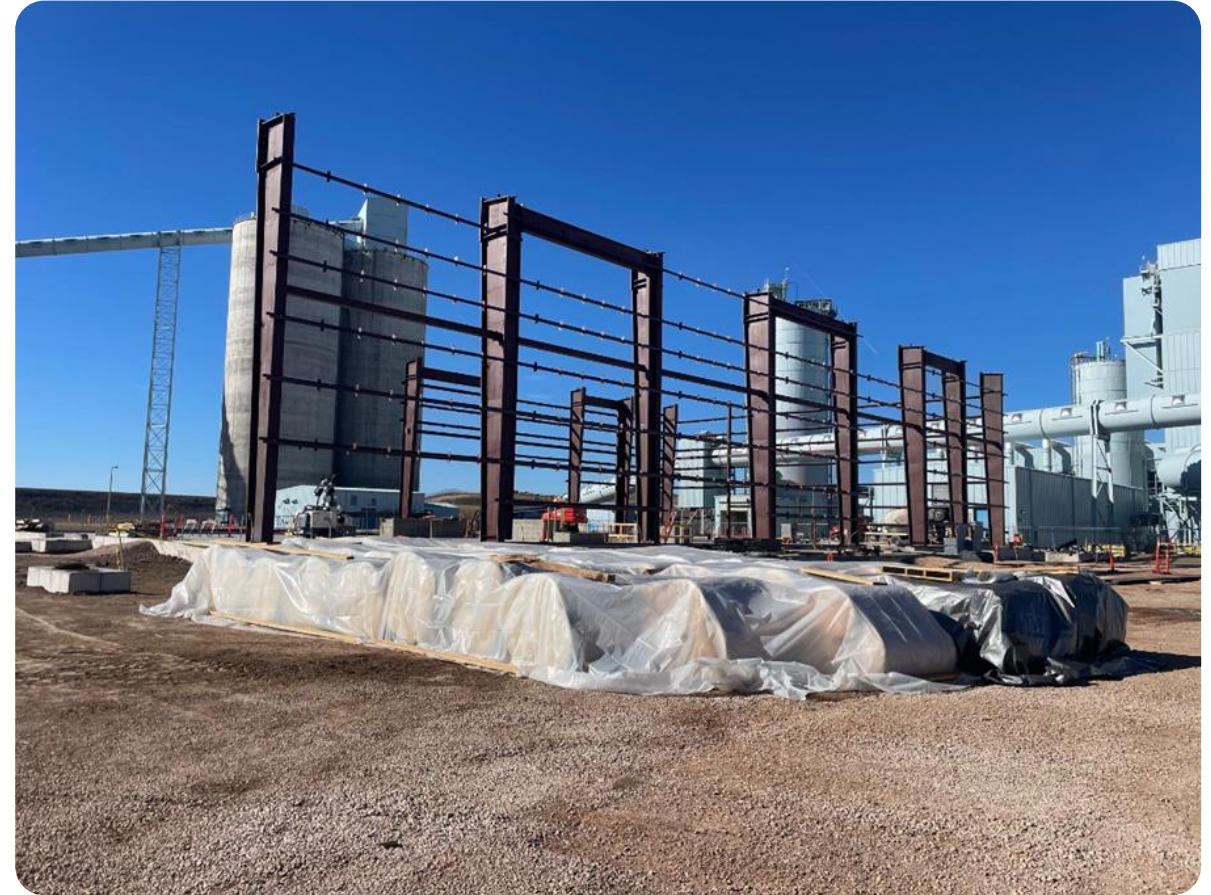
Steel members for the building are erected
