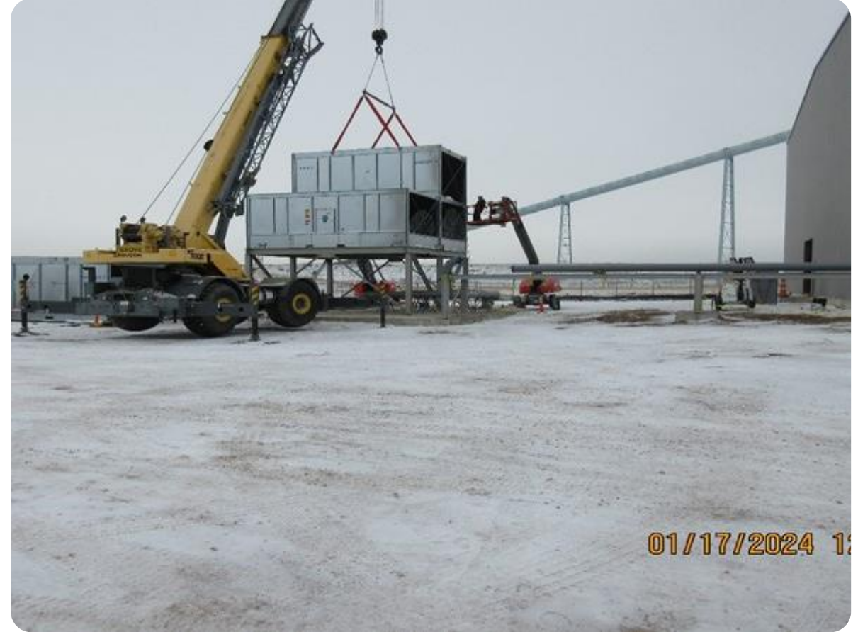
Evaporative Cooling Tower
