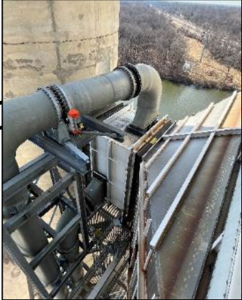
Flue Gas Ducting Tie-In
