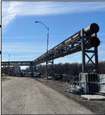
Flue Gas Ducting Bridge
