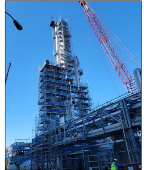
Columns erected on-site
