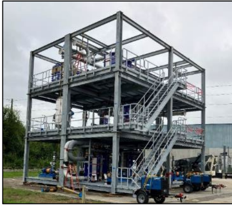
Modules at fabricator shop
