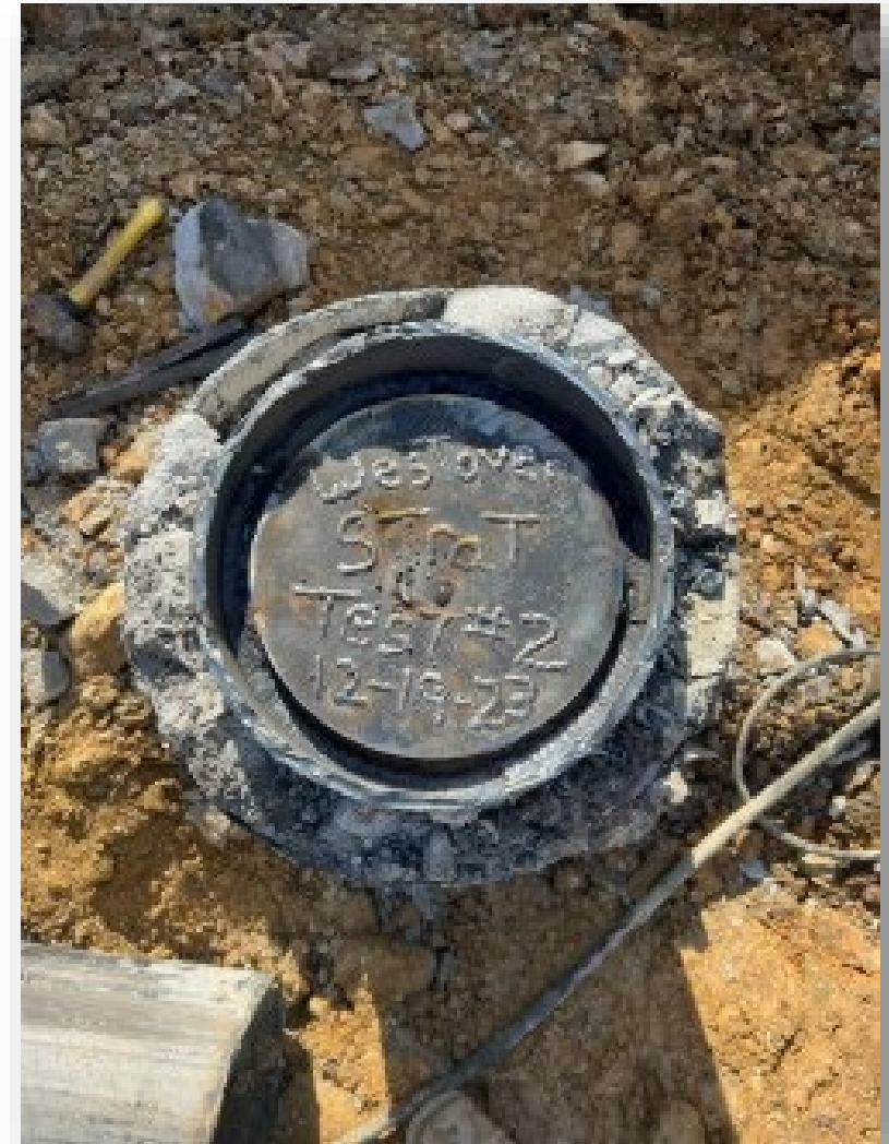
Photograph of the OASIS well site after reclamation and the well head fully plugged prior to burial
