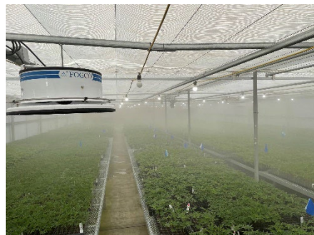
(3) Fogger/Misting system with reciprocating fans, linked to water lines
