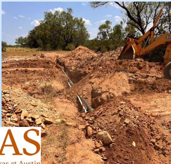
(12) Backfilling the trench
