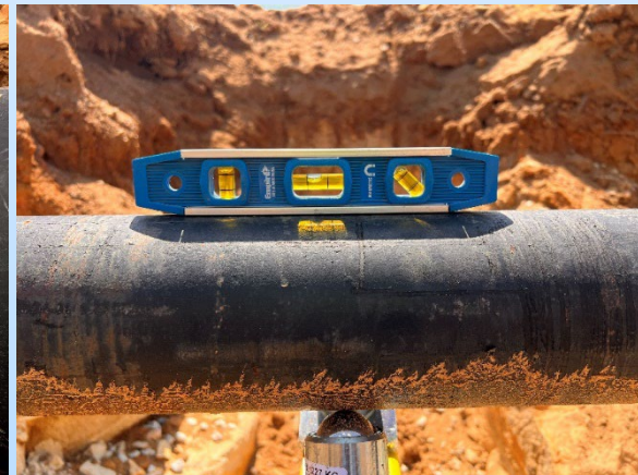
(6) Height adjustment - Inclination Toward Tank
