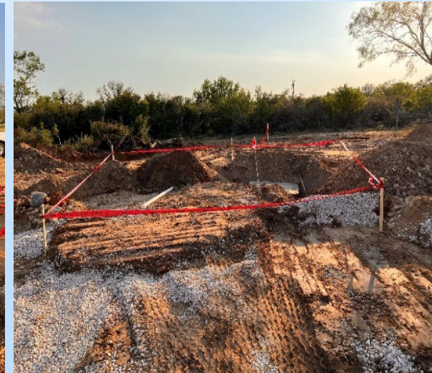
(13-14) Installation of safety signs and ribbons around the tank area
