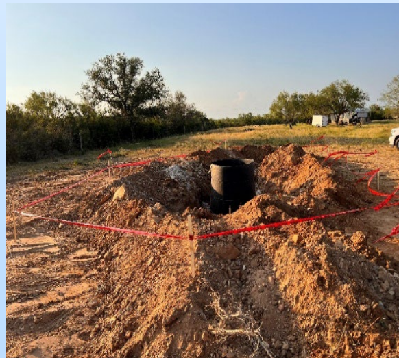
(13-14) Installation of safety signs and ribbons around the tank area
