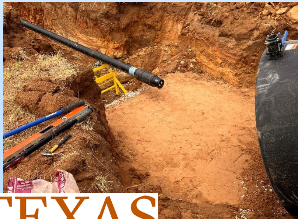
(5) Base Preparation for Tank
