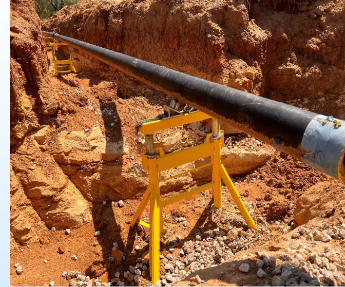
(7-8) Injection Pipe Assembly
