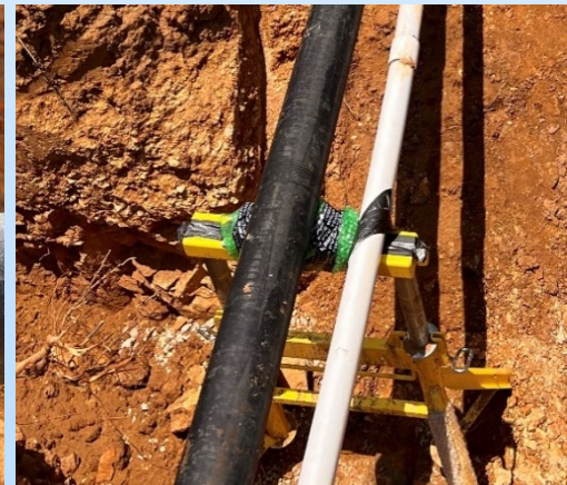
(7-8) Injection Pipe Assembly
