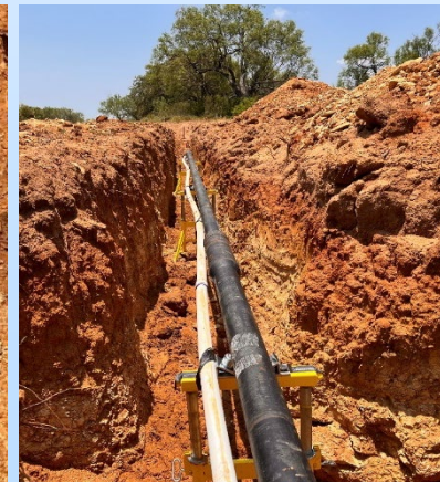
(7-8) Injection Pipe Assembly
