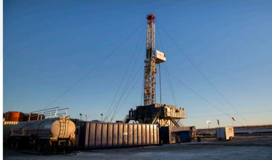
Test Well Drilling
