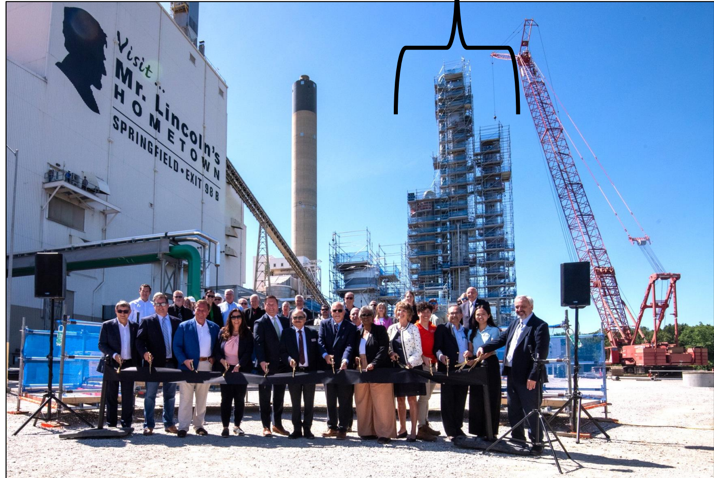
Ribbon-cutting ceremony for Carbon Capture Large Pilot Construction Site, DE-FE0031581
