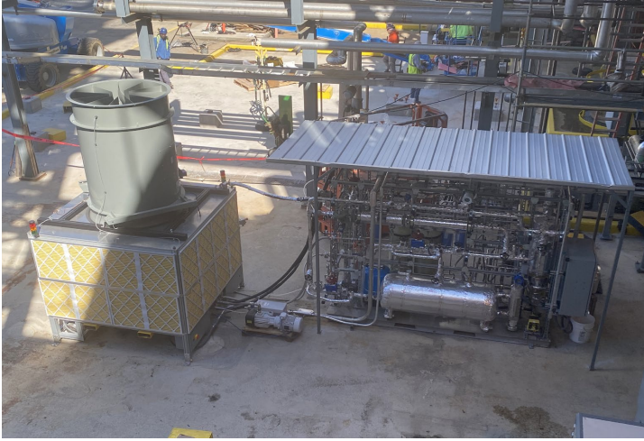
SN1: NCCC, Wilsonville, AL March 2023 to July 2024
