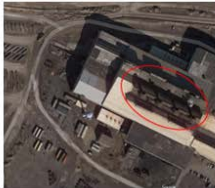
Tie-in to Waste Heat system
