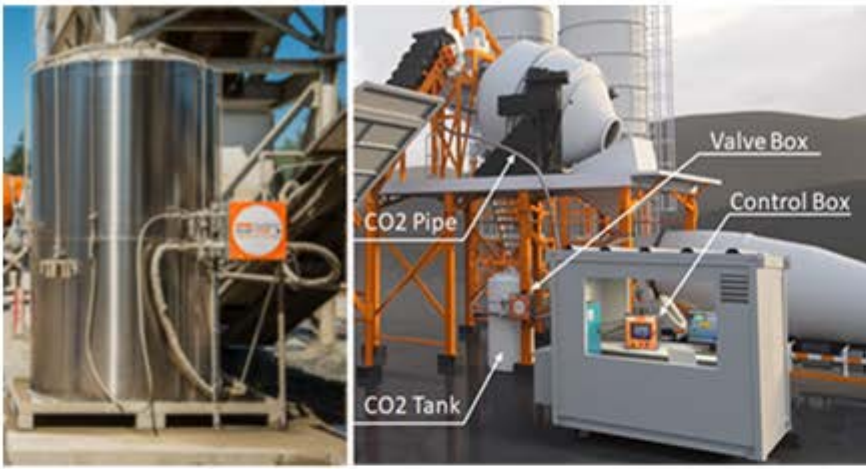
CarbonCure's retrofitted equipment into concrete plants
