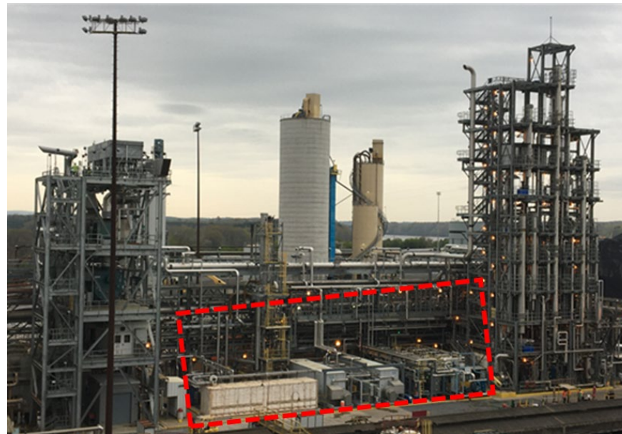
NCCC Pilot Bay Test Area
