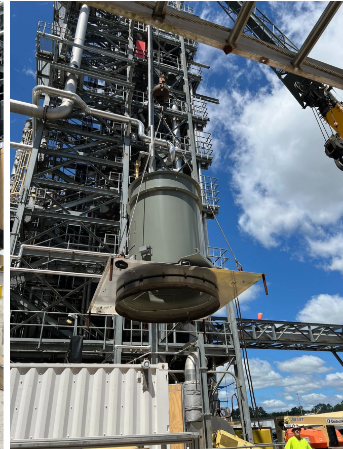
DAC-100 + Supporting Skids Decommissioning on July 8 th -12 th
