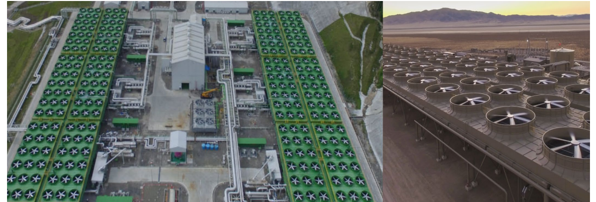
Air-cooled geothermal plants: 330 MW plant in Sarulla, Indonesia (left) and 27 MW plant Tungsten Mountain, Nevada (right Source: Ormat Technologies)
