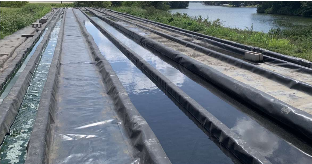
Larger Raceways Operated with Flue Gas Integration
