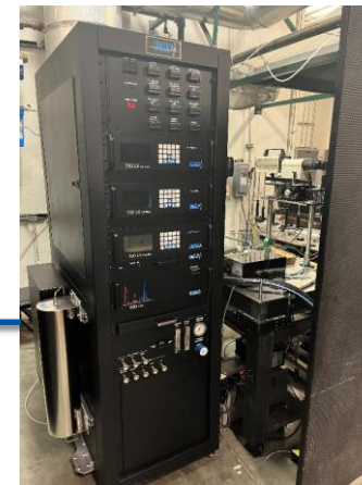
Water cooled Sample Line
