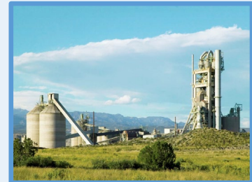
Balcones Cement Plant, New Braunfels, TX
