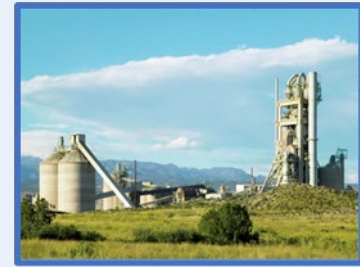
Balcones Cement Plant, New Braunfels, TX *
