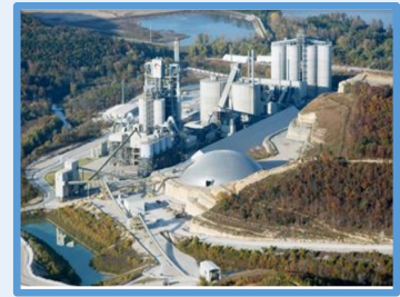
Holcim Ste. Genevieve Cement Plant Bloomsdale, Missouri
