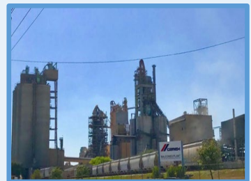
LafargeHolcim Cement Plant Florence, CO
