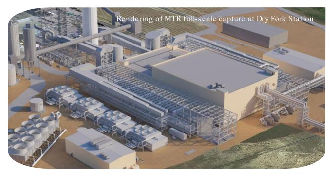
MTR and S&L recently completed a FEED study of full-scale capture at the DFS coal power plant including an AACE class 2 cost estimate
