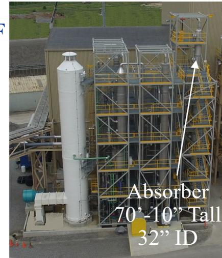
UK Small Pilot Evaluations with 14 & 4 vol% CO<sub>2</sub> Flue Gas by Dilution with Air
