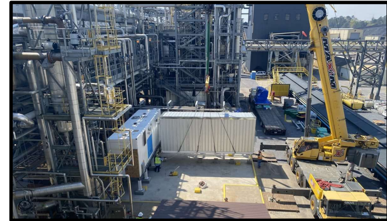
Initial Skid Placement at NCCC 3/16/23
