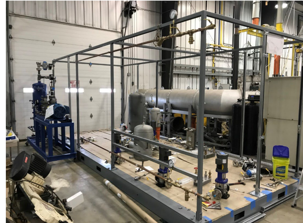
Test Skid Construction
